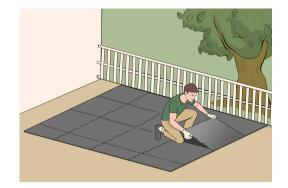
Start laying out the panels according to the layout diagram. "Staging" the panels allows them to acclimate to the ambient temperature as well as the adjacent panels. This also allows different crews to stay busy: one laying out panels and one snapping them together.
